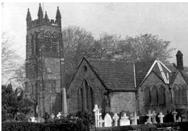
Photograph: 1976. St. Nicholas Church, Church Road, Halewood, was built using sandstone excavated from Woolton Quarry.
