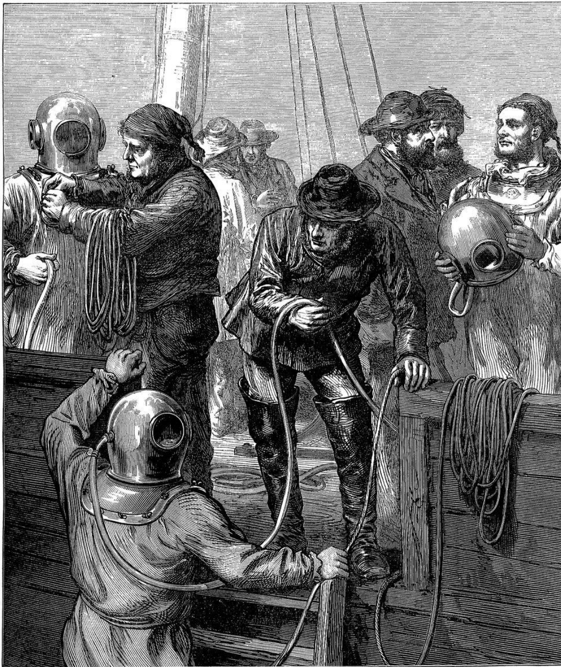
DIVERS PREPARING FOR WORK.
