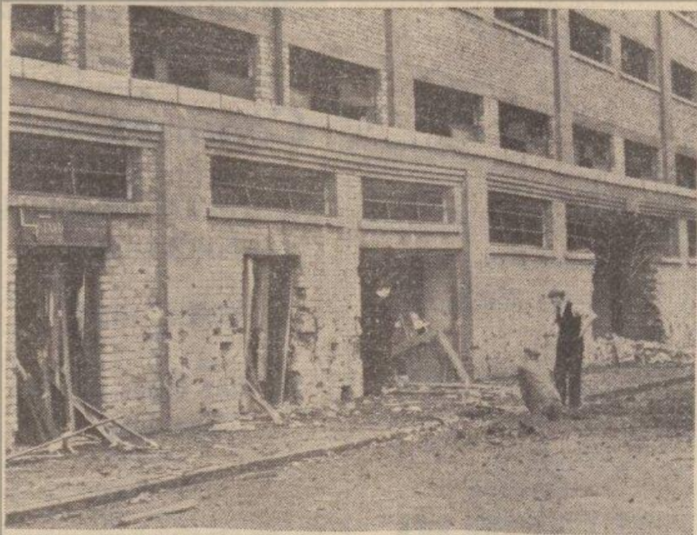
The rear of the stand of a well-known football ground, which was damaged during an air raid on a North-West town the same night.
